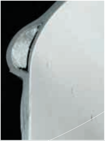
Jets and air track of domestic spa – note (inset) how air track is moulded into shell and therefore inaccessible for cleaning
